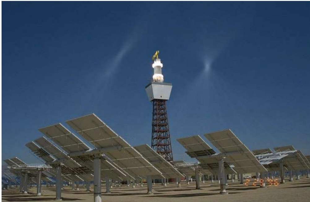
Figure 5: 10 MWe Solar Two power tower demonstration facility with molten salt receiver and storage at Barstow, California (Courtesy of SunLAB)
